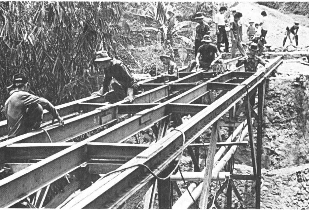
A passenger train at the Jakarta Railway Station Courtesy M. Rachmana Achmad Rural bridge construction in Jawa Barat Province Courtesy Indonesian Department of Defense and Security
